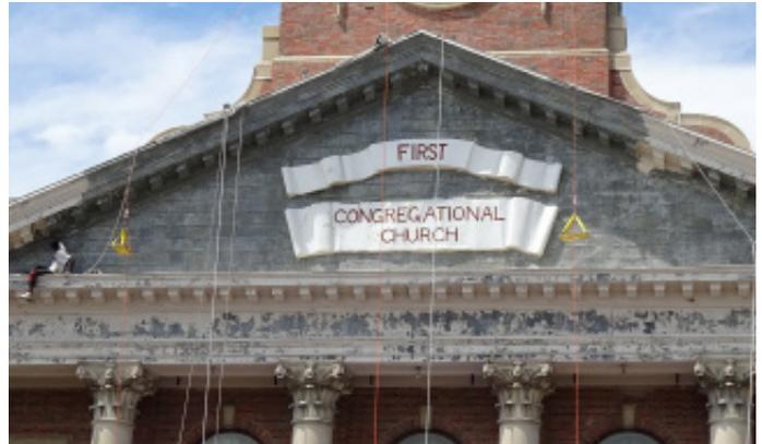
Workers from Inspired Heights, Inc., of Rockford, Illinois have been scraping lead-based paint from the roof and balustrade of the church since 2014. **Above left:** In early June 2015, workers suspended from ropes began removing paint from the church facade. **Above right:** By the beginning of August, much progress had been made. The scraped surfaces will be primed and painted. **Below right:** A worker dangling from a harness waved from his perch on the small tower.
