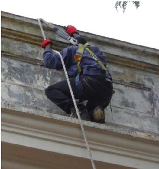
Throughout the summer, workers have been scraping lead paint from the balustrade prior to priming the surface for new lead-free paint. They are part of a crew from Inspired Heights, Inc., of Rockford, which provides church and steeple repair and restoration. Workers wear masks to keep them from inhaling small flakes of lead, and they wear harnesses to prevent falls. The lead removal has taken longer than expected, pushing work on the steeple and front of the church into 2015.
