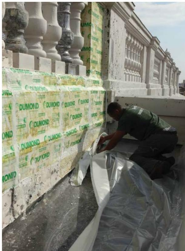
Above: On September 18, Morris, a member of the Inspired Heights crew, pressed strips of lead-removing paper onto the metal balustrade. After a time, the paper can be peeled off to reveal a clean surface. The procedure is ineffective in freezing temperatures, so work on this will cease as soon as the temperature drops below 32 degrees.
