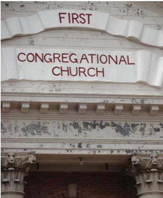
Left: A view of the facade of the church shows flaking paint clearly visible above the columns
