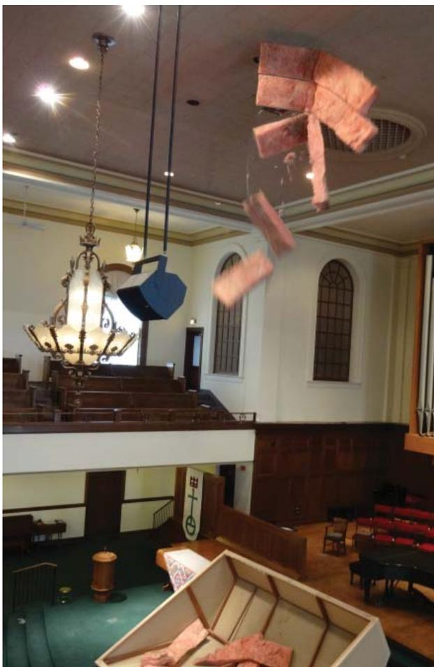
**At left:** Once the box was safely down and the horn and speakers were lowered, there remained hanging strips of insulation that had served as sound baffles. One by one, the insulation strips were released from their chicken-wire enclosures and dropped to the floor below. Then the old items that had clung to the ceiling for decades were carted off. **At right:** A hydraulic lift was needed to allow the painter to apply blue sealant and cream paint on the high ceiling of the Sanctuary.
