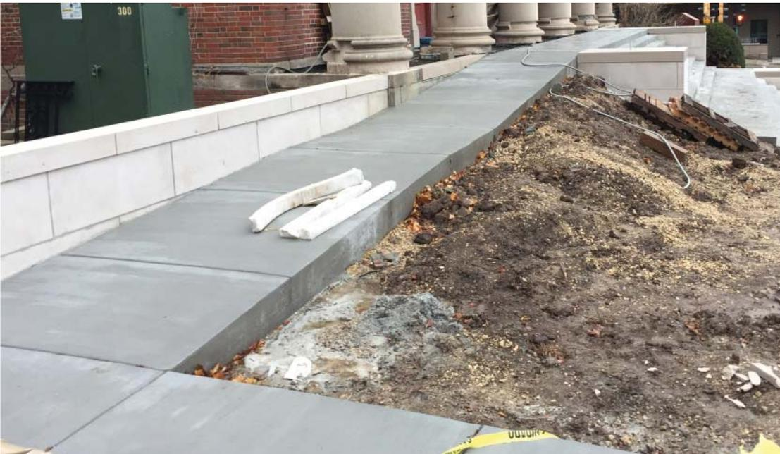
**Left:** In mid-November, concrete was poured for the new ramp which will make the front entrance fully accessible for the first time. All the concrete work on the stairs is finished except for the top landing, which can't be done until the bottom pieces of the limestone columns are installed. These pieces are being fabricated by the stone supplier, and should be ready soon. In the meantime, the only building entrances open are Lathrop Street, University Avenue, and Garden.
